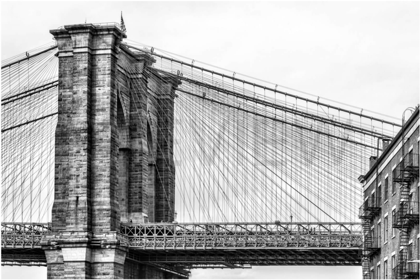
SUSPENDE GOthic STYLE Taken from DUMBO, this photograph of Brooklyn Bridge makes me want to climb to the top of its tower.
